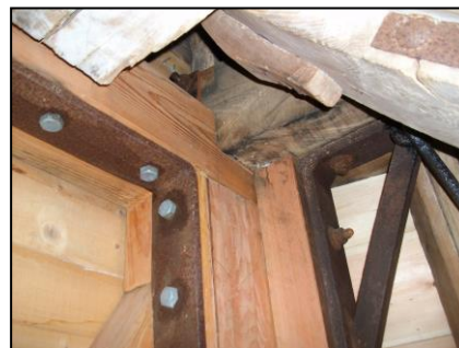
Above: Reinforcing brackets fitted to the top of the left breast corner post. The earlier cast iron bracket (1925) to the right supports the end of the weatherbeam. The new wrought iron bracket on the left supports the junction of a new timber corner post and upper side girt installed in 2015.
