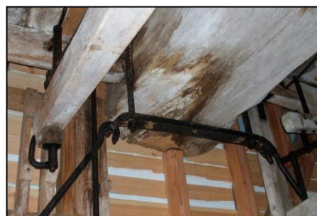
Above: Clamps on the end of the crown tree providing attachments for the diagonal tension rods that resist sagging at the front and rear of the mill body.
