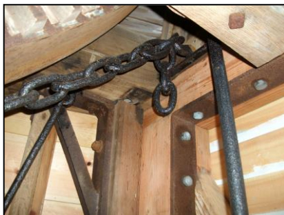
The picture left shows the fixing chain and connecting rod of the brake at the front of the stone floor.
