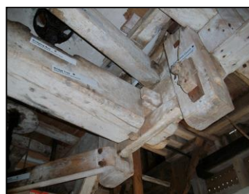
Underside of the bridge tree which supports the tail runner stone that can be seen above, its end mortise supported by a pair of hangers and cross bar. This is all original oak. Note the wedges used to retain the bridge tree tenon.
